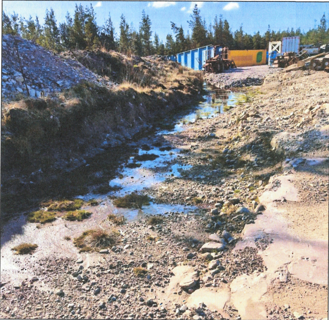
Plate 1-7. Artificial Field Drain located East of the Site (AWN, 2025)
