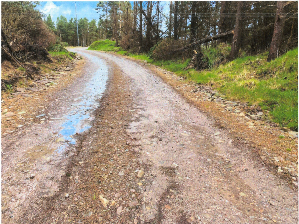
Figure 2. Gravel access road leading to site.
