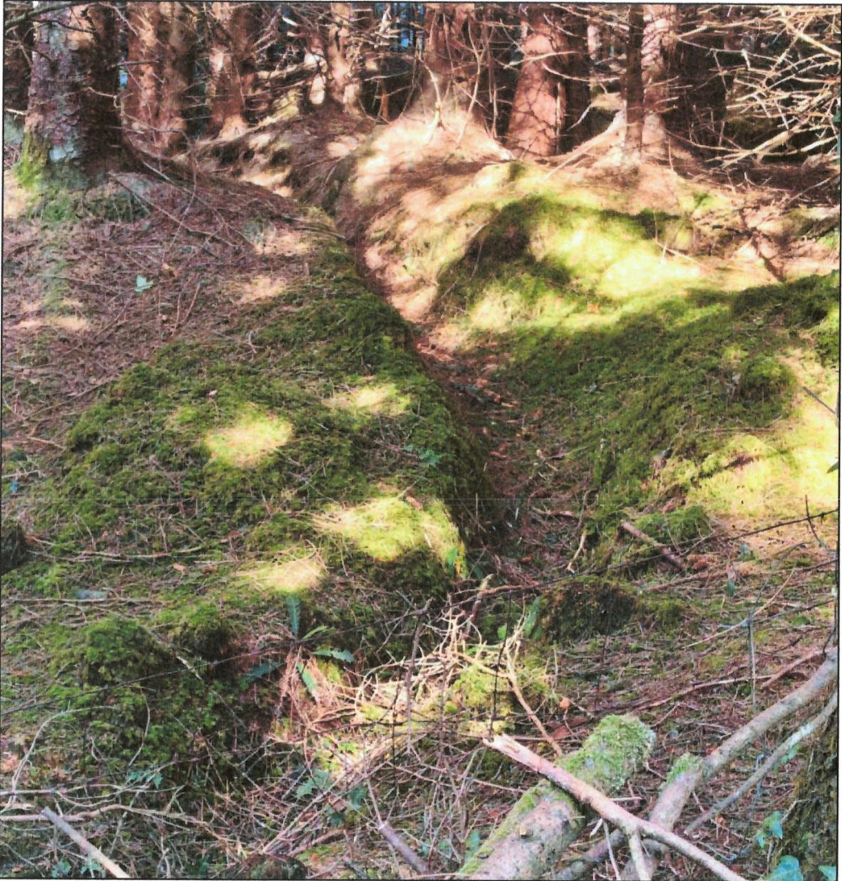
Plate 1-6. Seasonal Surface Water Drain East of the Site towards L 54213 (AWN, 2025)
